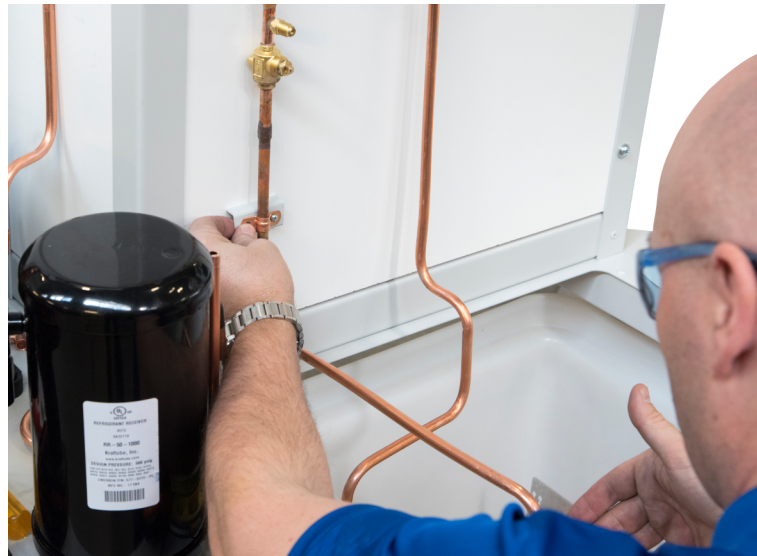
Figure 22. Technician installing spacers.
